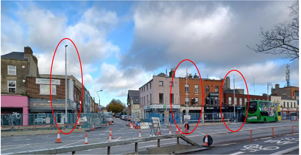
Fig. 2 – Embellishments yet to be installed (bottom of Fairview Avenue Lower)
